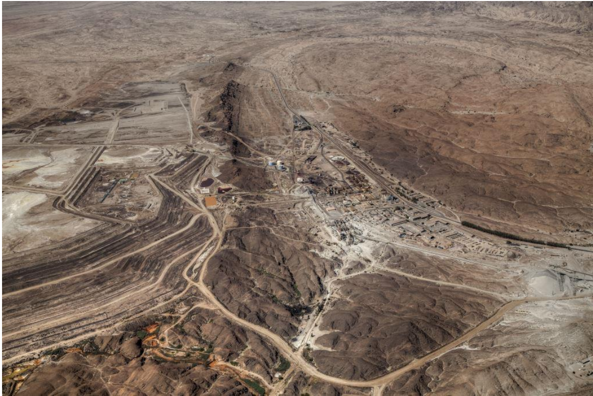
Figure 8: Rössing TSF with seepage appearing at the bottom toe of the dam. The view is towards the North (photo by André Terblanche)
